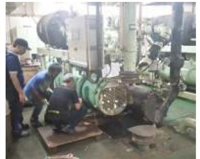
Vessel Name: KM. Kelud | Job Scope: AHU Coil Replacement
